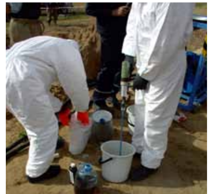
Preparation of epoxy
