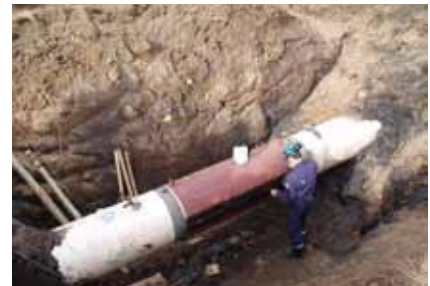
Quality control of sleeve welds
