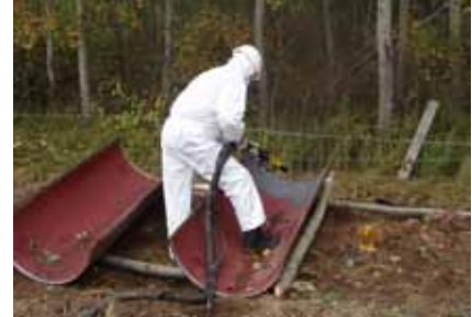
Grit blasting of metal half sleeves
