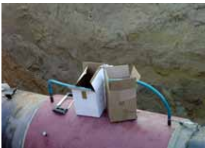
Monitoring of sleeve filling with epoxy
