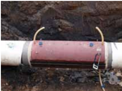
Sleeve prepared for filling with epoxy
