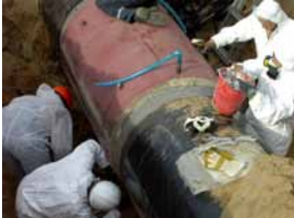
Sealing of pipe ends with fast curing agent
