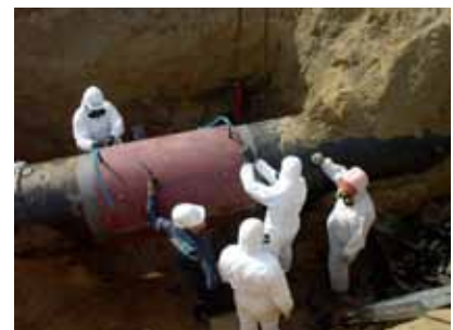
Adjustment of annulus gap from 0.2 to 1.6 in. (5 to 40 mm)
