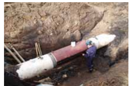
Quality control of sleeve welds
