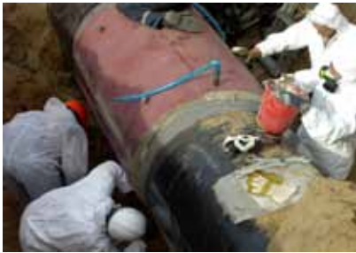
Sealing of pipe ends with fast curing agent
