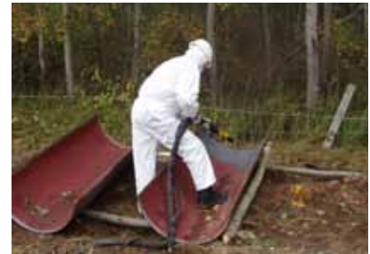
Grit blasting of metal half sleeves
