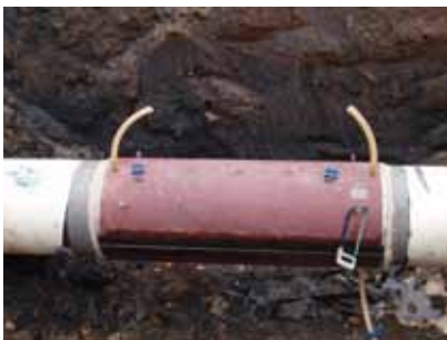
Sleeve prepared for filling with epoxy
