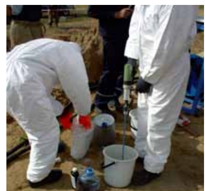
Preparation of epoxy
