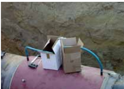
Monitoring of sleeve filling with epoxy
