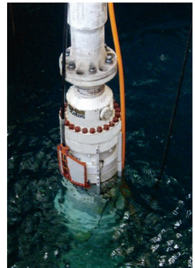
The successful installation of an API-certified submerged RCD in a riser and in tension is an industry first for this technology.
