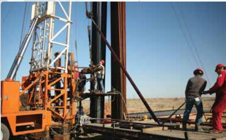
The *MetalSkin* cased-hole liner can be easily installed with a workover rig. No high-volume pumping equipment is required.
