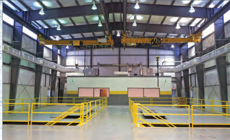
Our new testing lab features two underground bunkers, measuring 50 ft long x 20 ft wide x 15 ft deep with steel deck plates, to provide safe testing parameters for our accommodated test load frames.
