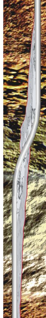
4. Shifted casing ready for repair
