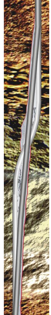
5. Repair liner installed, ready for cement productions
