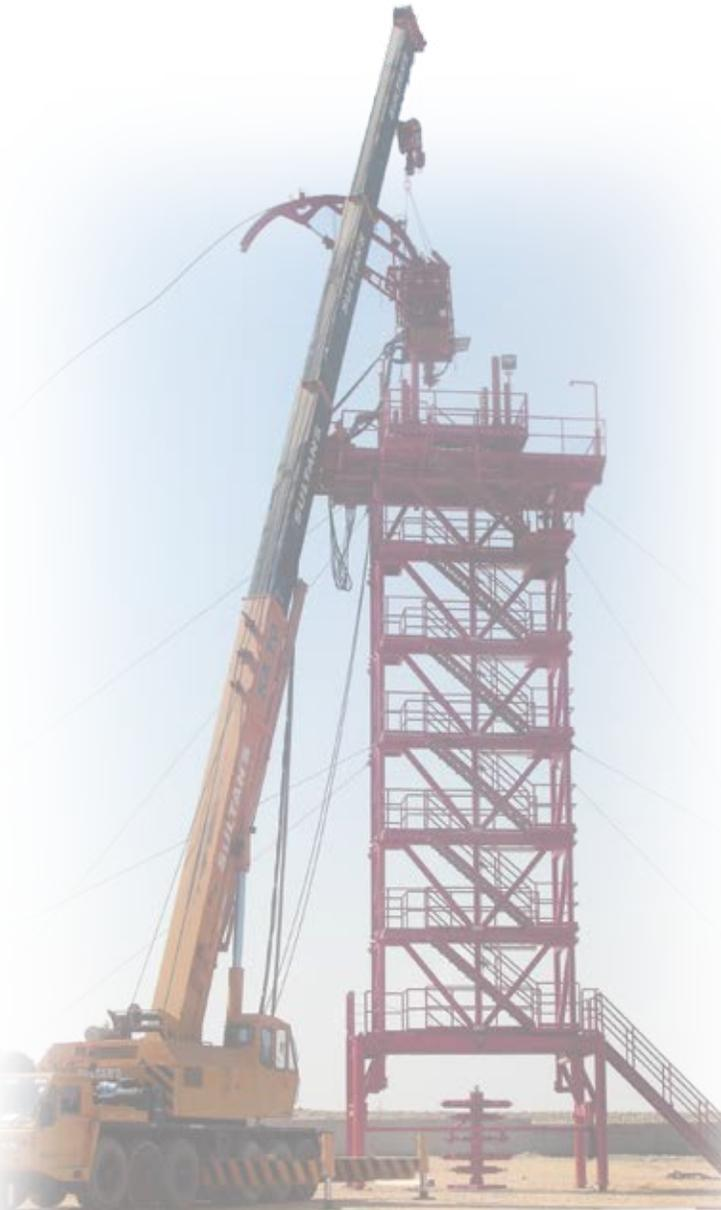
A coiled-tubing drilling rig being constructed in Algeria.
