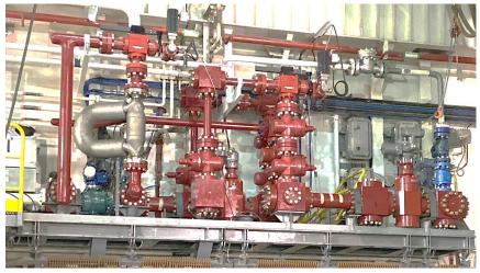
The Victus MPD manifold, choke, flowmeter, and piping occupied a compact footprint on a specially fabricated walkway to avoid interference with lifting, cantilever skidding, or deck operations.
