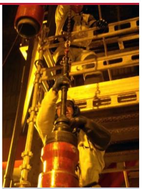
Weatherford's 7-in. damaged bore safety valve, part of the *Renaissance* system, enabled the operator to reestablish well integrity after multiple attempts at sealing standard insert valves in damaged seal bores. This was the first 7-in. WBD installed globally and the first *Renaissance* application in Norway.
