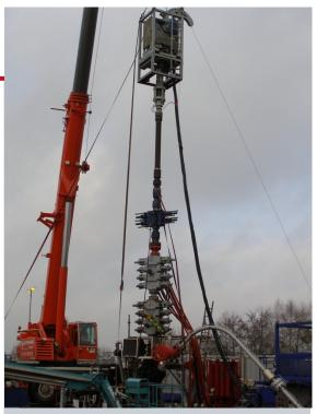
The Weatherford Renaissance WDCL system efficiently replaced a damaged TRSSSV in a sour-gas well. Using equipment that can withstand corrosive downhole conditions, this operation helped the client avoid the expense of major workovers while restoring production to optimal levels.
