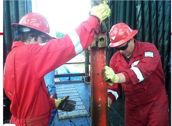
Weatherford fast-track whipstock supervisors prepare the *QuickCut* casing exit system for deployment to 18,241 ft (5,560 m) in an onshore gas well.
