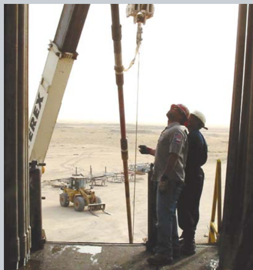
Workers examine the shallow-angle QuickCut casing exit system as it is readied for the well.
