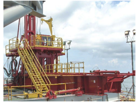
The Weatherford pulling-and-jacking unit situated on the wedge deck during decommissioning operations at the wellsite in the Gulf of Mexico.
