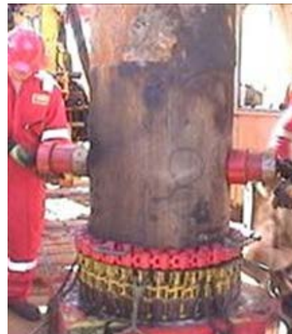
Weatherford devised a plan to remove casing and conductor from four low-producing wells on different platforms. The above picture shows boring in the first section.
