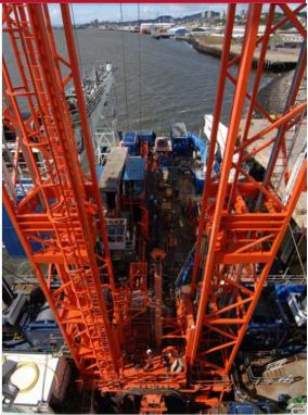
The ram rig lowered Weatherford's M24 cutting tool through the moonpool down to the seabed and cut the casing. The *MOST* tool pulled the cut casing and wellheads to the surface.
