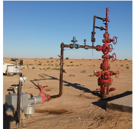
The Weatherford plunger-lift system overcame the liquid loading problems in the abandoned well and restored production.
