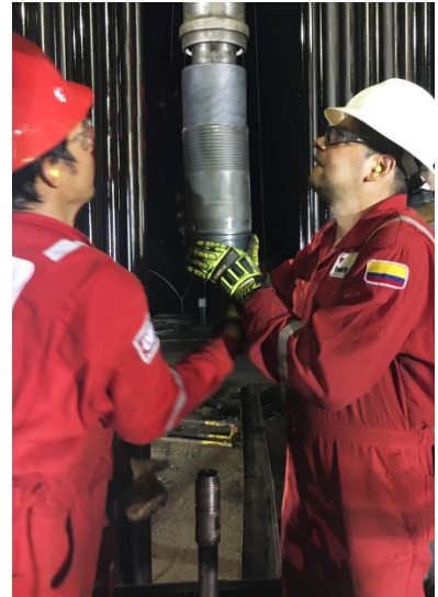
Working with a small workover rig, Weatherford casing integrity specialists in Colombia run the X-SPAN casing patch downhole to repair a section of damaged casing.
