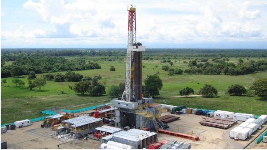
Weatherford provided integrated project management and support services for the entire operation.
