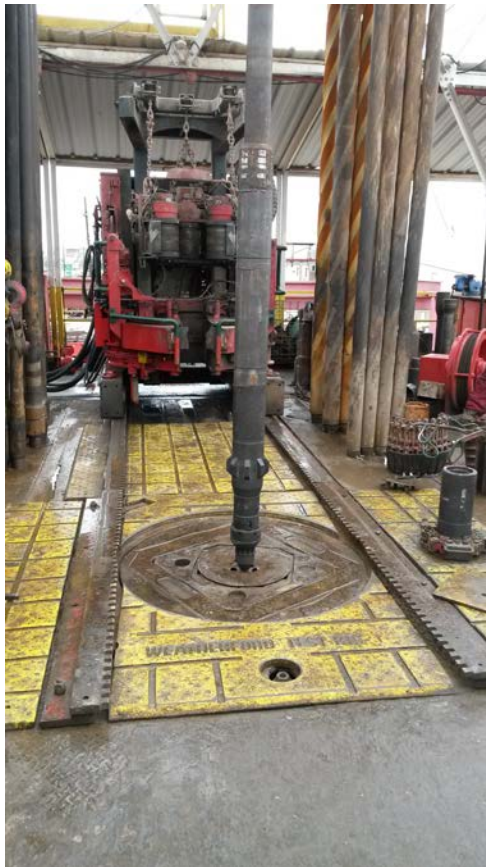
The photo to the left shows the retrievable DwC WRRD at the wellsite.
